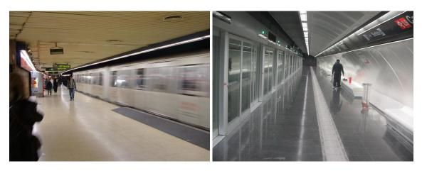
Figure 9: Platform design for both old (left, open platform) and new (right, platform screen door systems) subway lines in the Barcelona Metro system.
